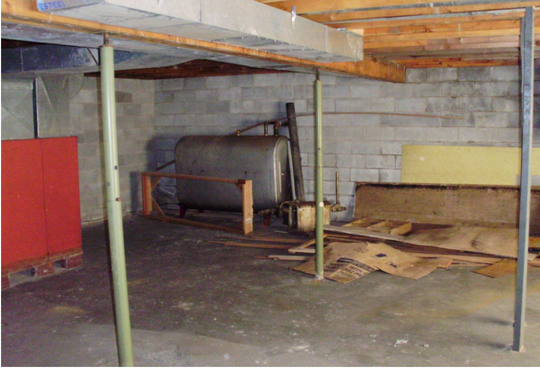
Photo 1: Basement, 900 L fuel tank in NE corner. Appears to be empty.
